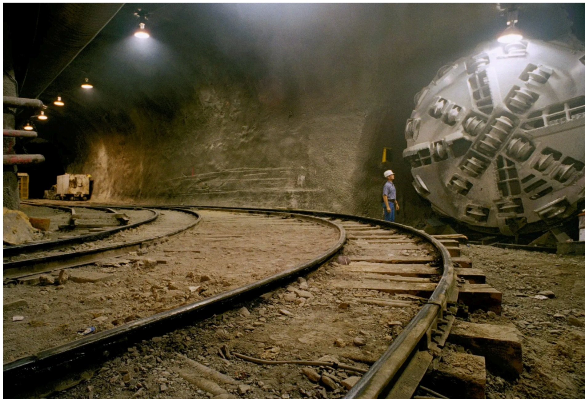
A tunnel of the Superconducting Super Collider project in 1993, which was abandoned by Congress. Ron Heflin/Associated Press
